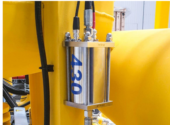
In-line Tan Delta measurement
